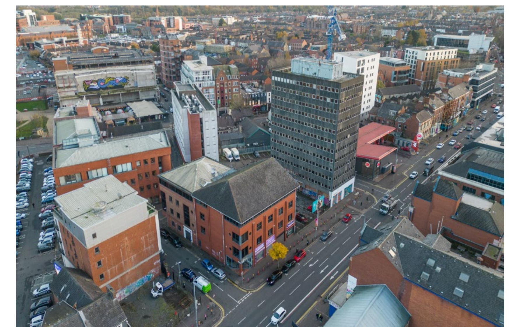
EXISTING FANUM HOUSE
